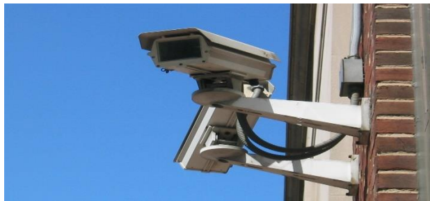
With an overt CCTV camera, the public (and offenders) can clearly see the surveillance camera and determine the direction in which it is facing.
