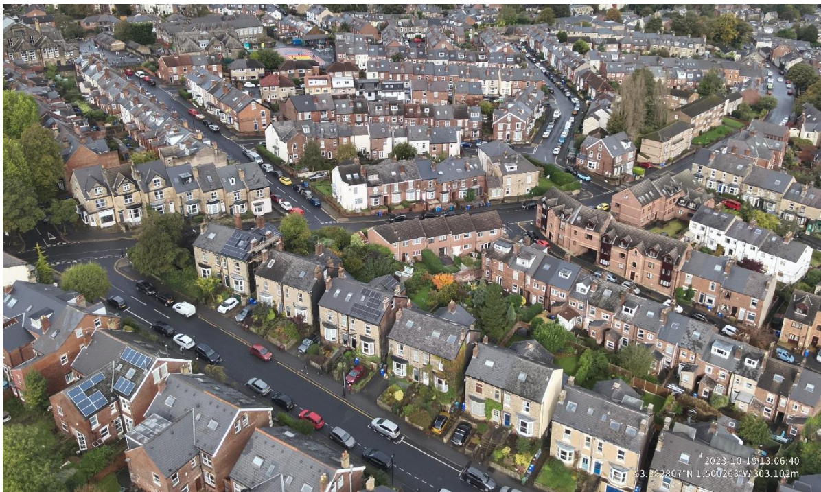
Figure 6: Photographs of same streets in the Crookes area from 1980 and 2023. On the first picture there are 53 cars parked on the road, in the second 133, an increase of 151 per cent
