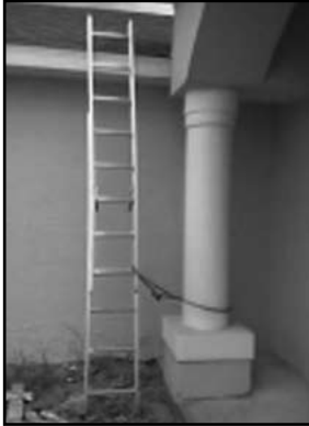
Example of target hardening of construction equipment.
