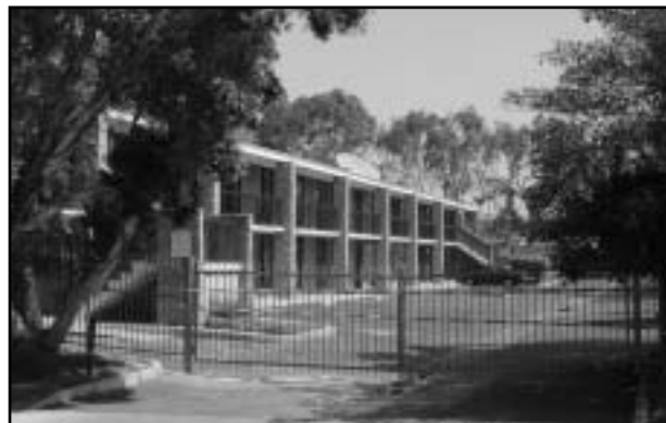
This motel fenced an unnecessary entrance/exit to reduce "pull-through" traffic.
