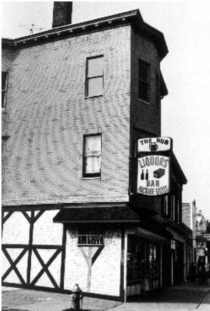
The Model Noise Ordinance recognizes the vertical and horizontal boundaries of a property line. A bar below an apartment is regulated by the Model Noise Ordinance, but not the State's Noise Control Regulations.
