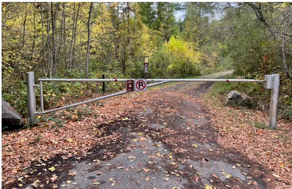
(a) Tubular gate preventing access to/from private road (lock receptacle on the right of the photo)
