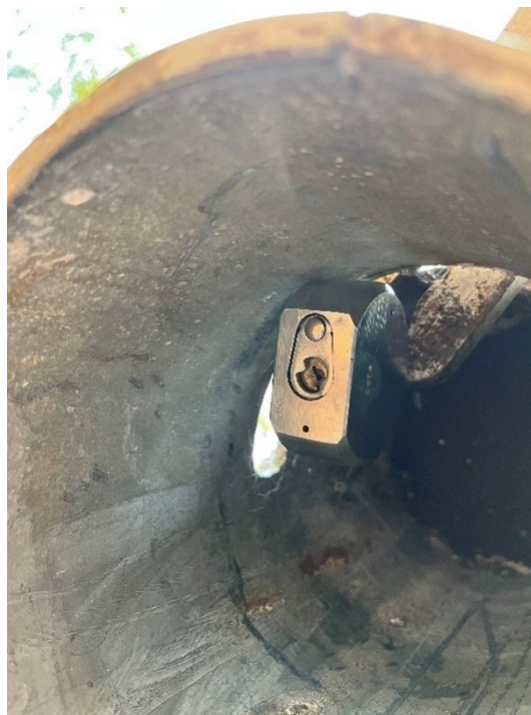
(c) View from below the lock receptacle
