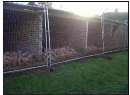
Demolition of garages
