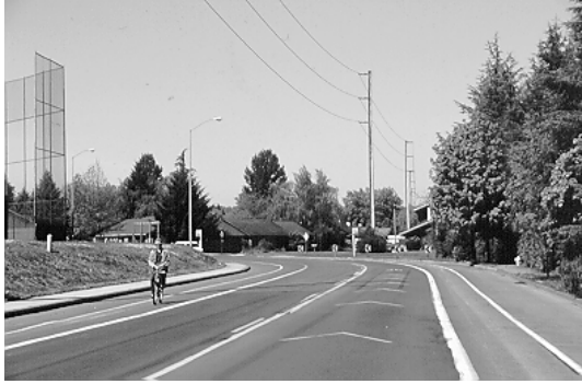
Figure 5.49. Transverse Markings on a Horizontal Curve. (Eugene, OR)
