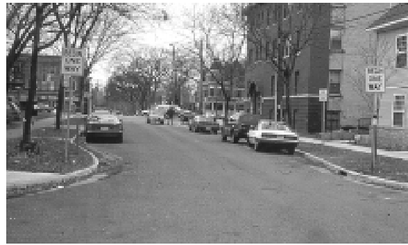
Figure 5.46. Short One-Way Section to Discourage Traffic Through a Neighborhood. (Minneapolis, MN)
