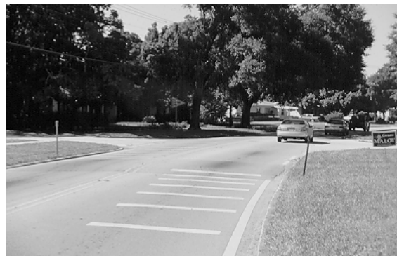
Figure 5.48. Transverse Markings on the Approach to a Speed Hump. (Seminole County, FL)
