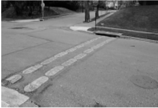
Figure 5.43. Intersection Jiggle Bump. (Dayton, OH)
