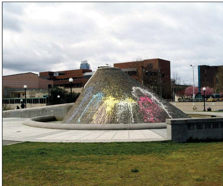
Figure 4 – Vandalism on the Cal Anderson Park Fountain, 3/30/08
