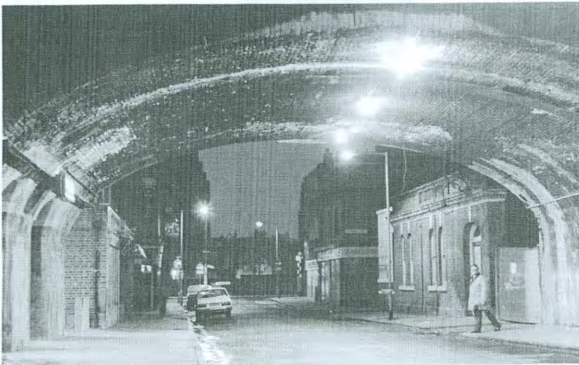
Railway Bridge : After
