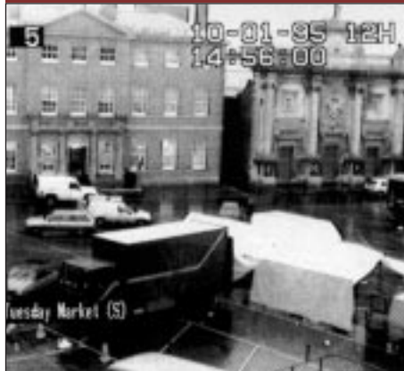
Figure 23 Two of King's Lynn's car parks also serve as market places. Note the camera can monitor activity outside surrounding buildings
