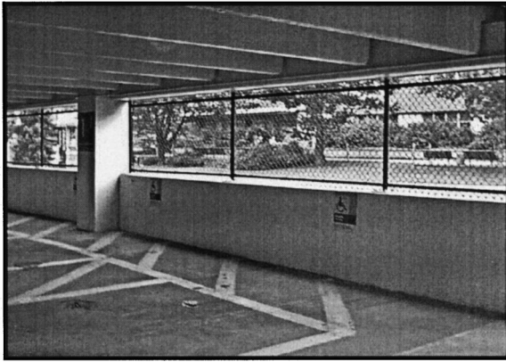
Fig. 5. Chain-link inserts in lower level parking garage wall openings
