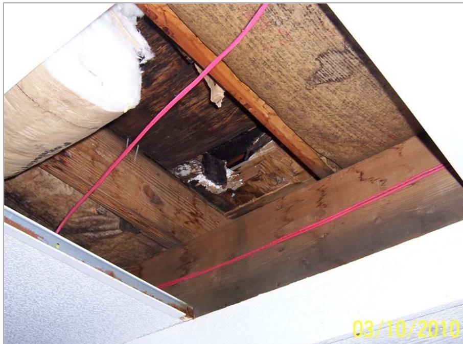
Figure 11: Note the rot and damage.
