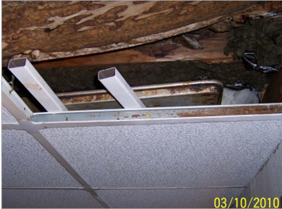
Figure 10: A cookie sheet catches rain water beneath a leaky roof.
