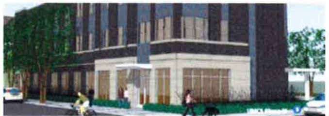
UMCS Phase III will be completed in 2012 and will provide a home for Milwaukee Bicycle Works and Community Pie
