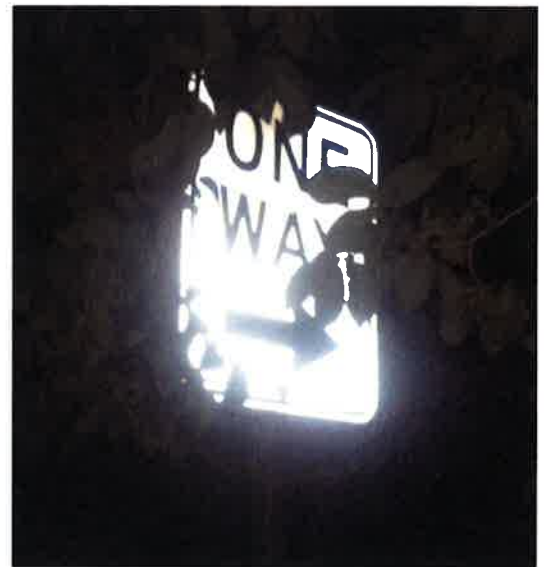
Signage was obstructed by overgrown trees.
