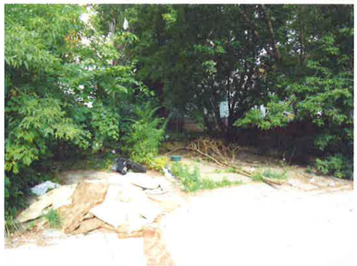
Concrete parking pad off of the alleyway that is overgrowth & a dumping ground.
