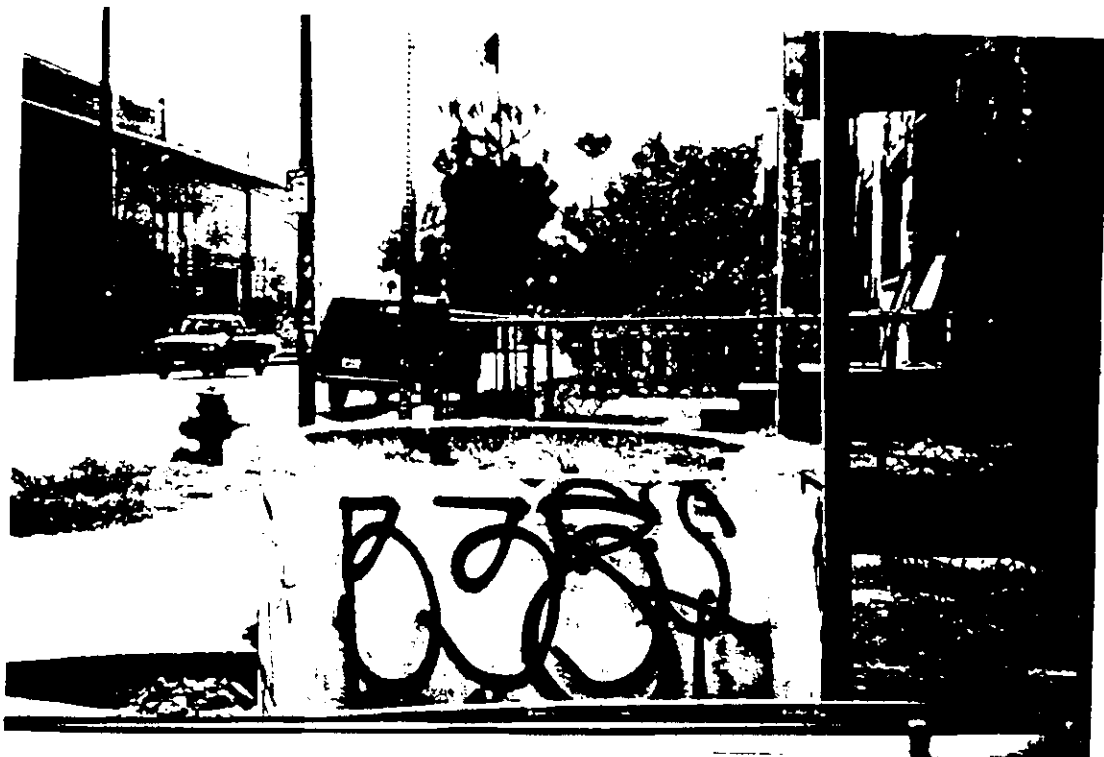
Shown Above: Cement planter used as trash can, with tree dead and gates removed
